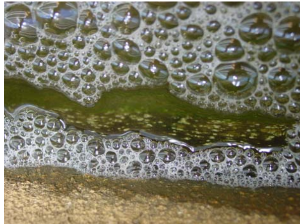
Figure 2 – Sediment in Cooling Tower Basin
