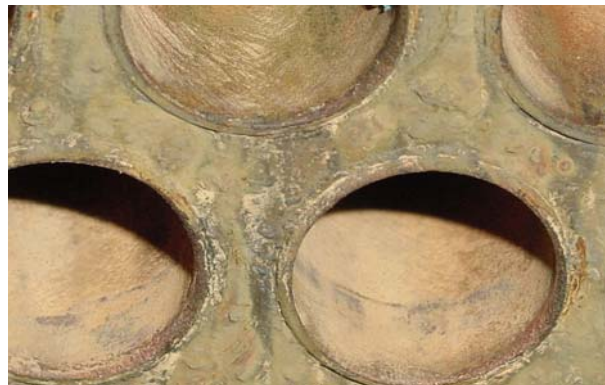
Figure 3 – Chiller tubesheet
